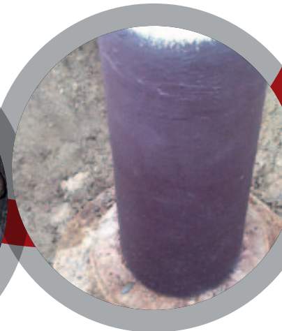
Repair of Thin Wall Defects
