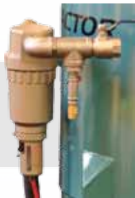
SMC 1-1/2" BSP Quality Filter on solid 1-1/4" Piping
