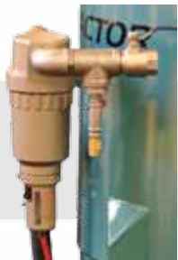
SMC 1" BSP Quality Filter on solid 1" Piping
